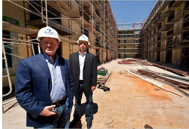
Frank Middleton, left, and Brian Pianca of Wood Partners, which is finishing the project.
